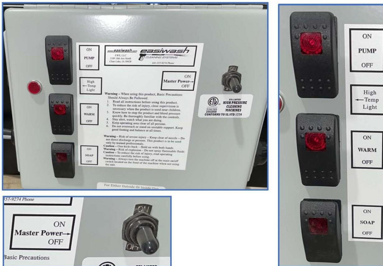
Before turning on power make certain the control box is wired for the proper voltage. [Power Unit – Final Install Instructions, page 2 of 4] of the Install Playbook. Measure incoming voltage from the building. If it's 215V or lower the red wire from transformer should be connected to L3 on contactor. If incoming voltage is over 215 V the orange wire from transformer should be connected to L3 instead of the red wire.
